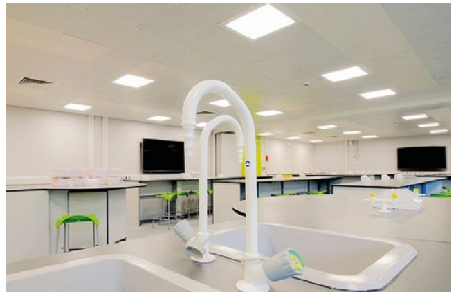
Figure 4: Installation of low-glare luminaires in IT rooms and science labs for Thornleigh Salesian College limited screen glare, delivered uniformity and optimal spacing to prevent shadowing, and provided adequate lighting for detailed tasks. The light delivered from the opal polycarbonate diffuser, CRI>80, CCT of 4,000K up to 120lmW -1
