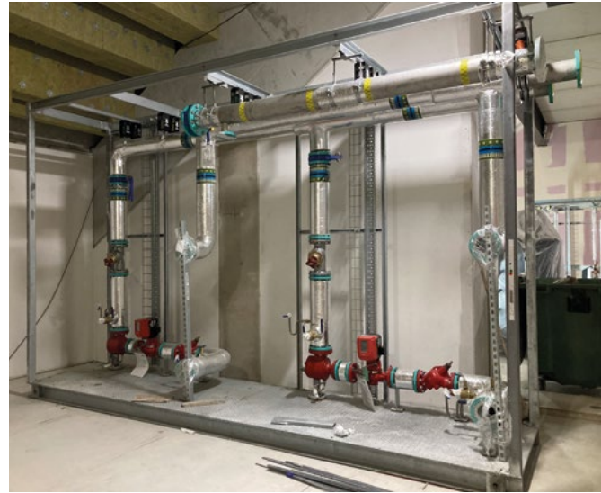
A plant skid manufactured in Laing O'Rourke's factory
