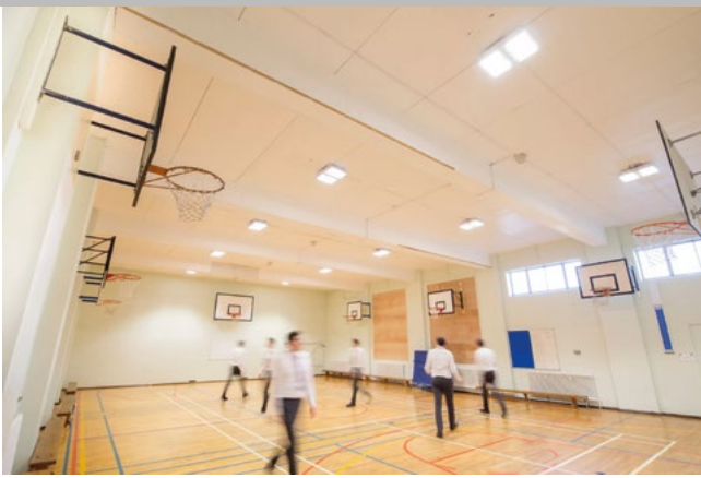
Figure 1: High-output luminaires (with wire guards) were used in the gym of Hastings College. These luminaires have a high output with a wide-angle optic. This LED module delivers CRI>80, CCT of 4,000K and up to 168lmW -1
