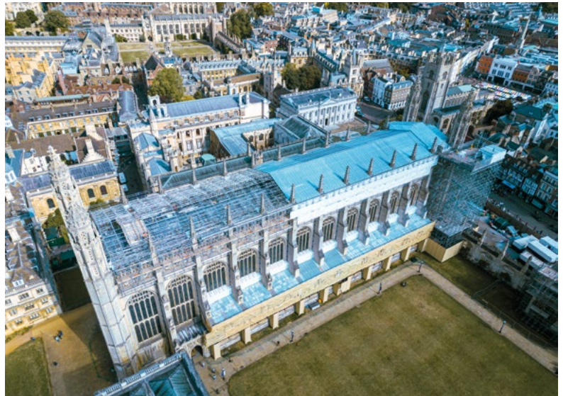
The shallow 25° angle of the roof pitch meant that the north and south slopes were suitable for PVs
