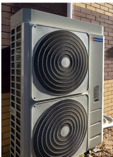
Figure 2: This is an example of a monobloc R32 air source heat pump with a heating SCOP of up to 4.48 (@ 35°C flow) and 3.31 @ 55°C – this particular range has outputs of between 14 to 70kW and can be cascaded to achieve higher outputs in larger installations (Source: Hamworthy)
