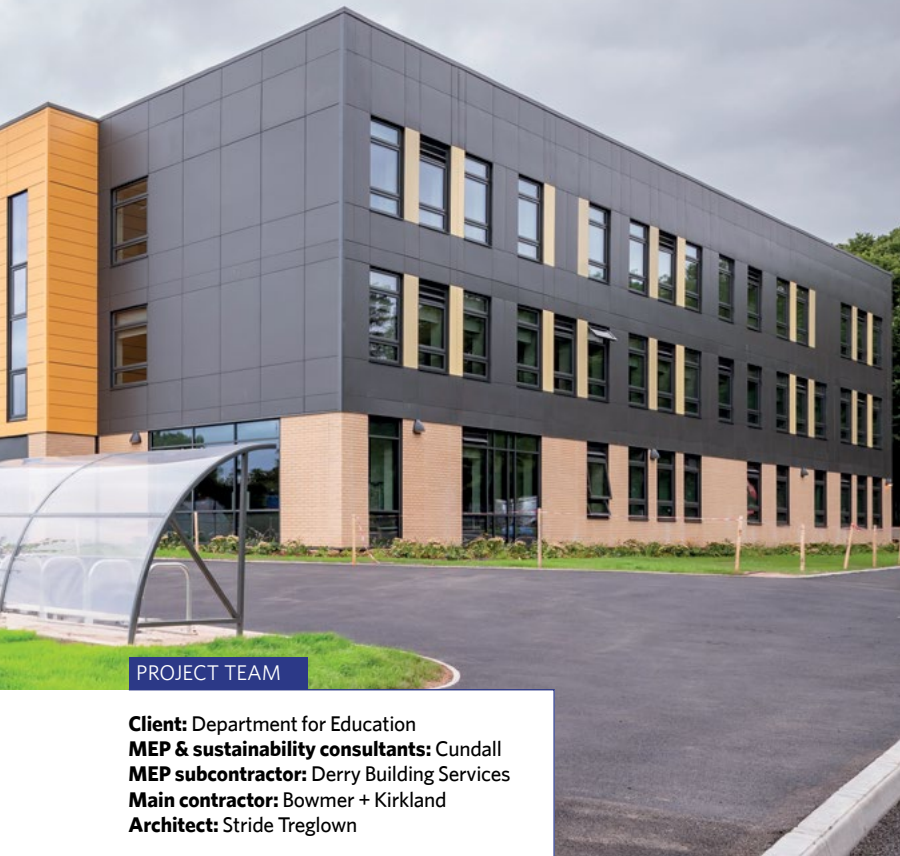
Left: The school's well-insulated and airtight façade features Innovare structural panels and high-performance glazing
