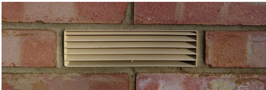
Figure 2: Examples of powder-coated steel ‘mechanical airbrick’ (Source: Titon)
