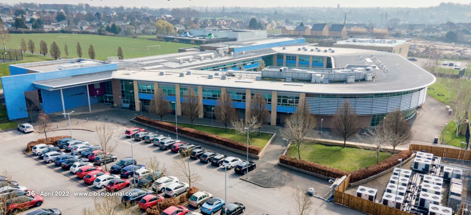
Bishop Young C of E Academy, one of the Abbey MAT schools. The air source heat pumps can be seen in the bottom right of the picture
