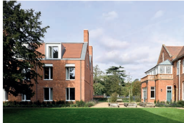
Left: The south elevation of Agar Grove, showing the balcony, which provides private amenity space and solar shading for summer comfort
