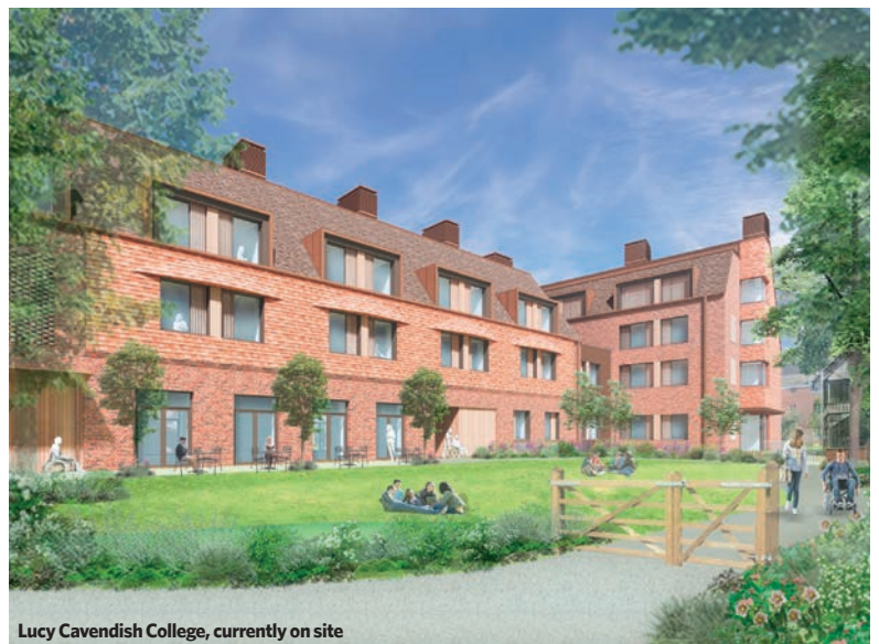
Lucy Cavendish College, currently on site
