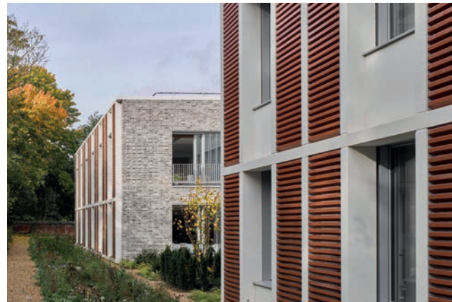
Two external characters, one low-energy approach: the Villa building (above top) and the Stephen Taylor building (above bottom) share the same low carbon cross-laminated timber (CLT) primary structure, all-electric energy system, and Passivhaus construction quality. The Villa building has a brick façade to complement the arts and crafts context it sits within, while the Stephen Taylor building has a precast concrete and brick façade, in response to the modernist architecture seen elsewhere in Cambridge.
