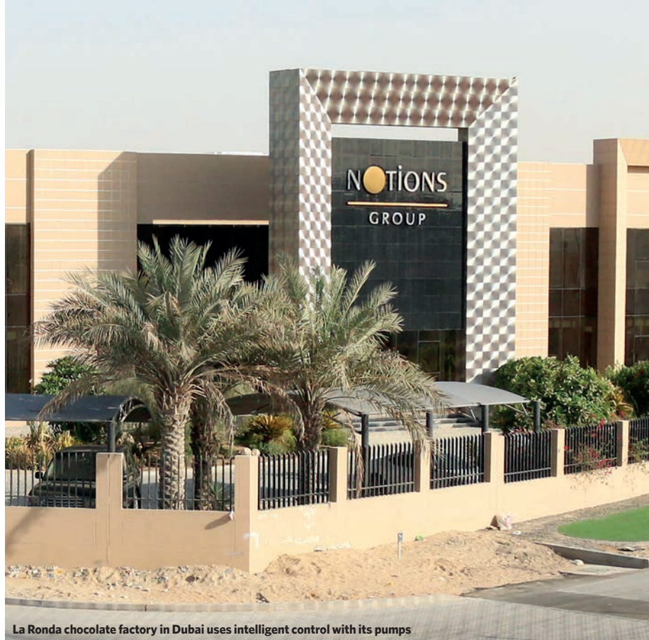
La Ronda chocolate factory in Dubai uses intelligent control with its pumps
