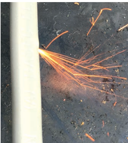
Development of a series arc fault within a cable sample
