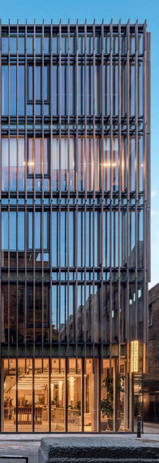
The louvre timbers are positioned vertically on the east and west façades and horizontally on the southern façade
