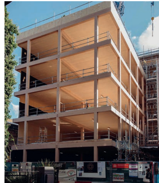
The floor slabs and staircases are all built from CLT
