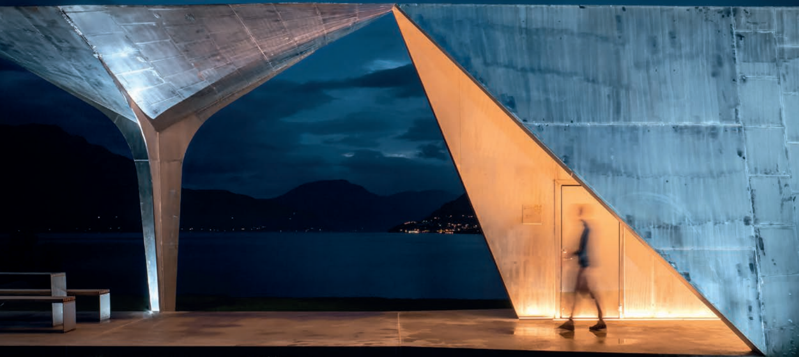
The roof and wall surfaces are made from 6mm-thick steel plates
