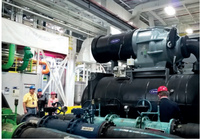
The chillers used in 22 Bishopgate underwent witness tests in Carrier's facility in Charlotte, North Carolina
