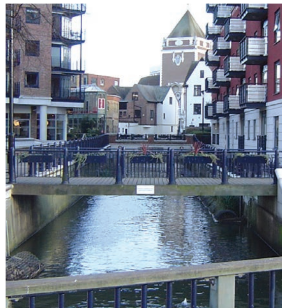
Thames Water flushes 69 million litres of clean warm water into the Hogsmill river in Kingston every day, as treated effluent
